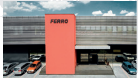
FERRO headquarters in Skawina
